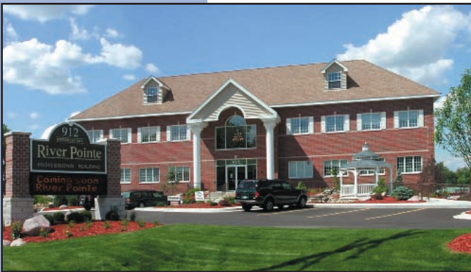
River Pointe – High Tech Medical Offices Fox River Grove, IL 51,540 sf
